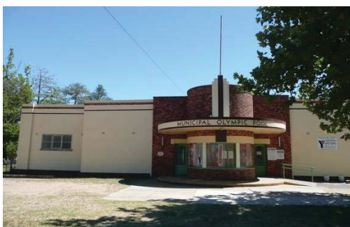
Maryborough Municipal Olympic Swimming Complex, 1940
