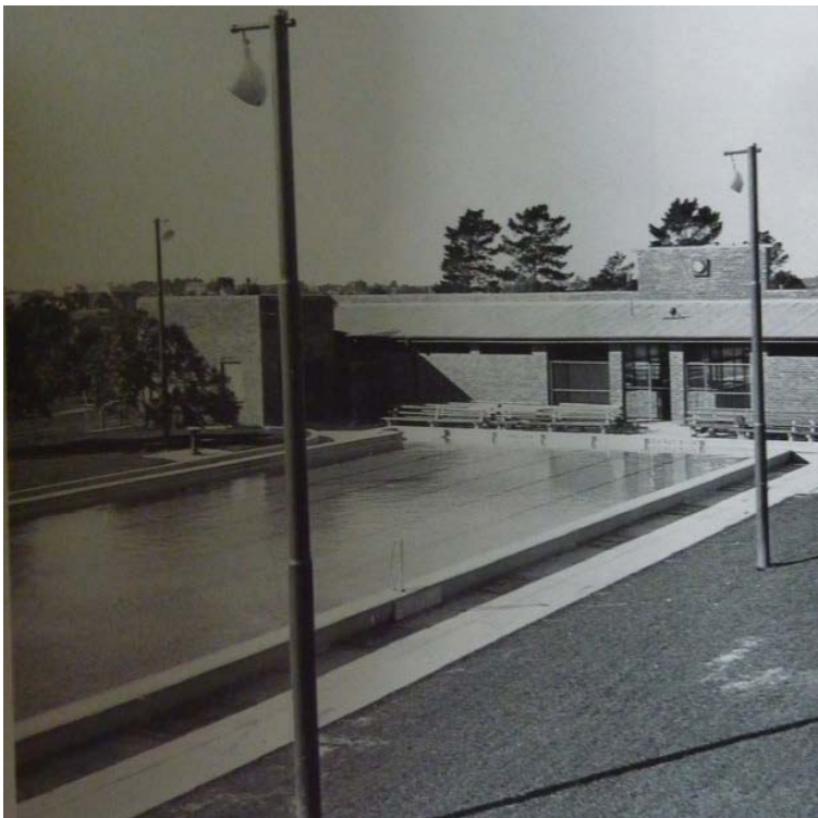
Swimming Pool soon after opening, from E Finlay & M Morgan, Those Were the Days, Box Hill in Pictures 1930-1960 , p 49; 1994
