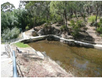
Hepburn Springs Swimming Pool, early 1930s
