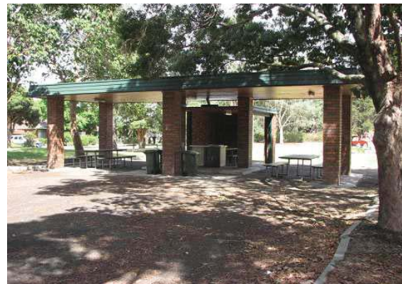
The former ticket booth/entry gate (1975) since converted into a public BBQ shelter
